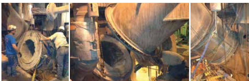
Refractory line high temperature expansion joint installation
